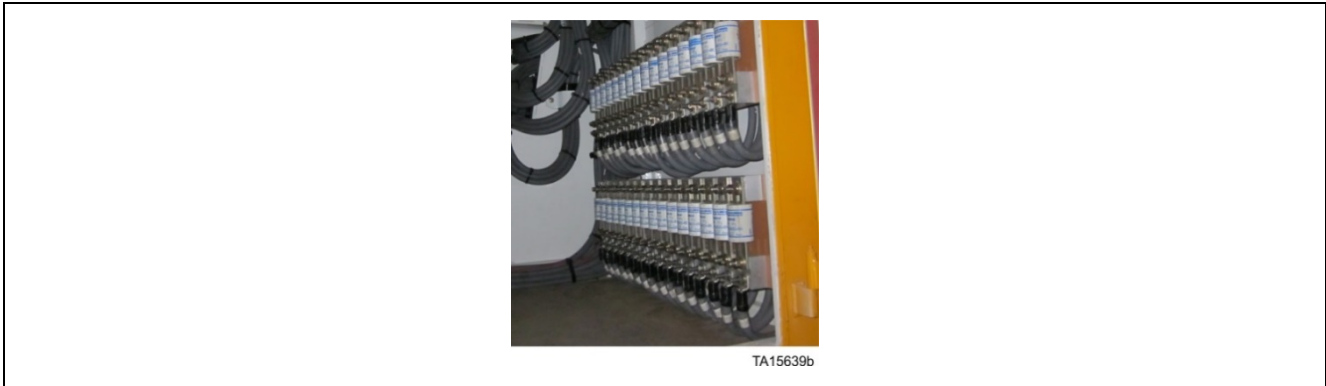
Figure 90. Fuse assemblies (L-2350 shown)
