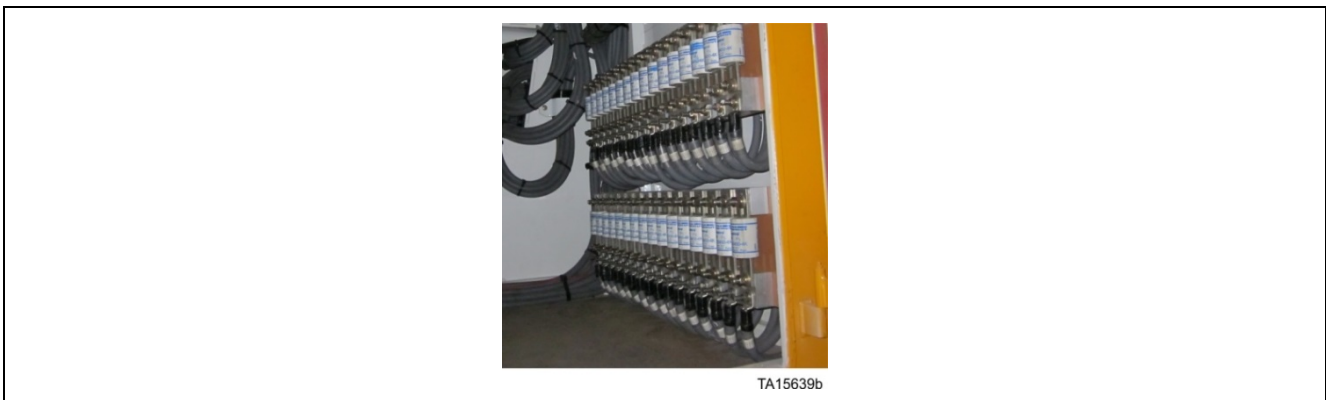
Figure 49. Fuse assemblies (L-2350 shown)
