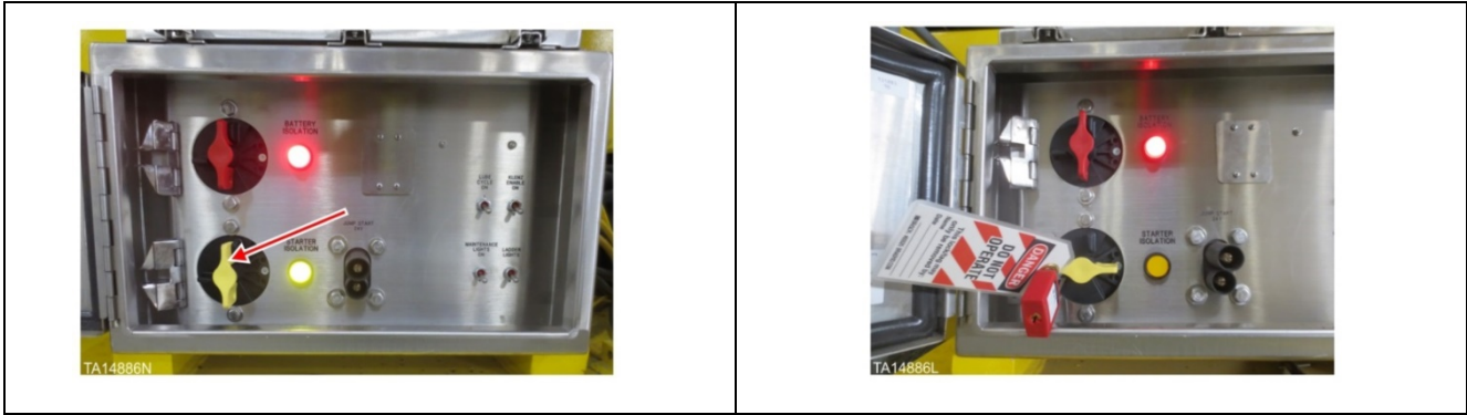
Isolate and lockout the starter
